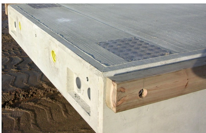
Concrete pontoon and perimeter timber fender detail.
